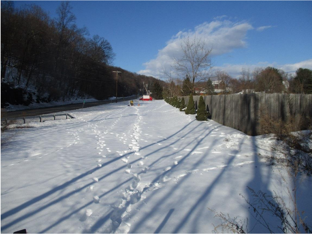
LANDSCAPING & FENCE ALONG ROUTE 9W
